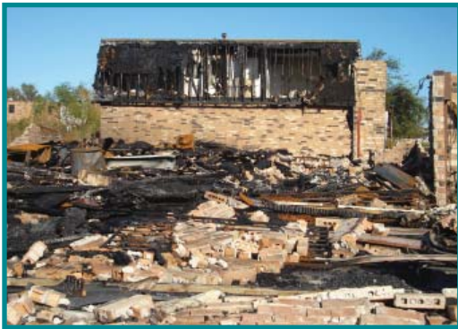
This wrecked home remains standing in New Orleans, three years after Hurricane Katrina.
