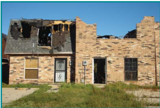
This home, one of countless others damaged by Hurricane Katrina, remains in ruins three years after the storm.
